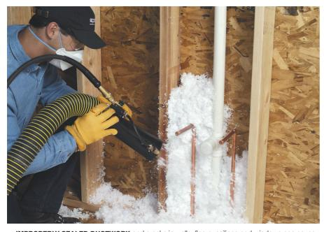
**IMPROPERLY SEALED DUCTWORK** and cracks in walls, floors, ceilings and windows can cause air leaks, allowing outdoor pollutants to infiltrate and compromise indoor air quality. Proper insulation, seen here, can seal up these openings without adding volatile organic chemicals like formaldehyde to the indoor air environment.
